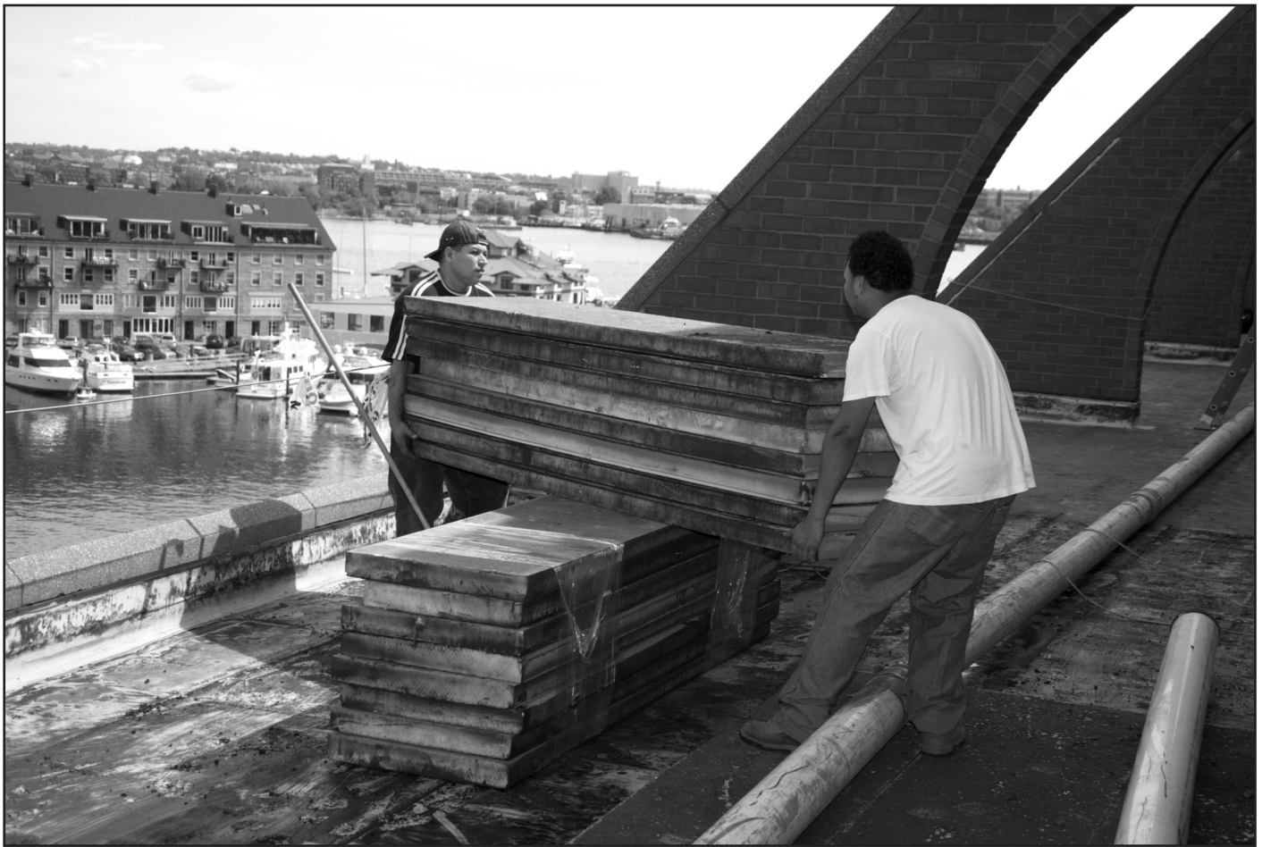
Figure 9 – Extruded polystyrene insulation being saved for reuse.
